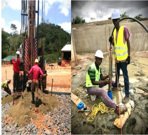
Borehole Redevelopment & Mechanization
