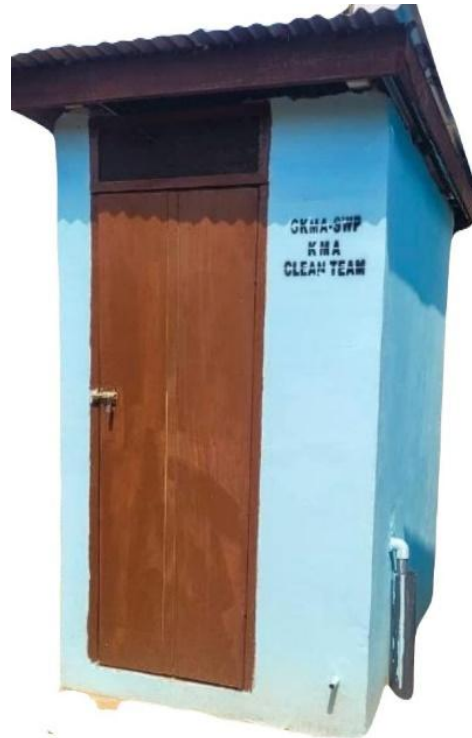
Bio digester Toilet
